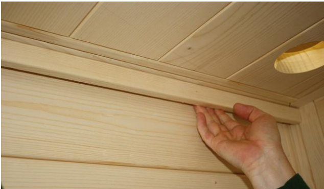
Obr. 38: Nalepenie LED pásov
